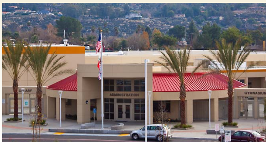
Hemet High Renovation Project—Admin Bldg 2011
